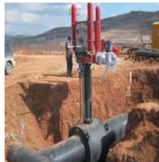
Welded body valve with extended stem
